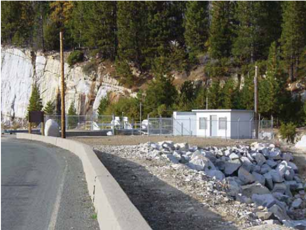
Photo J-3. View of safety fence surrounding the French Meadows Dam Generator Building.
