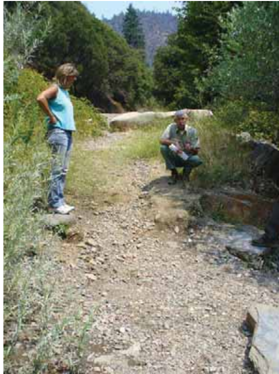
Photo L-3. Car Top Boat Ramp as viewed from lower part of ramp (7/23/08).
