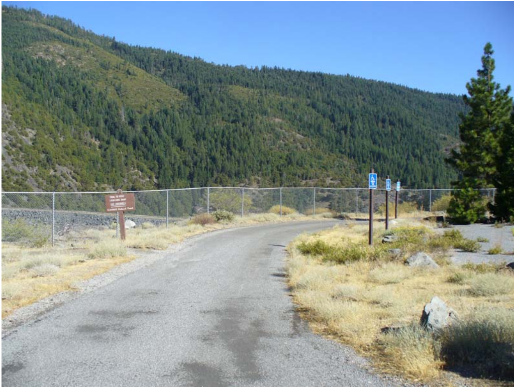
Photo E-2. View of barrier fence surrounding Hell Hole General Parking Area.
