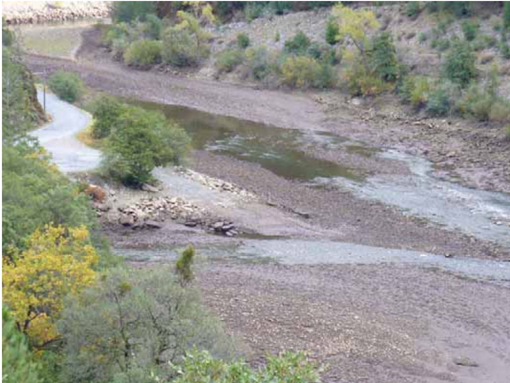
Photo L-5. Sediment removal access point on Ralston Afterbay. This site is not a Project recreation facility but is sometimes used to access the reservoir. (11/12/08).
