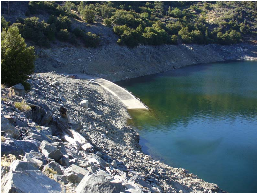
Photo B-4. Hell Hole Boat Ramp as viewed from Hell Hole Boat Ramp Parking Area (August 20, 2008, WSE = 4,568 ft)
